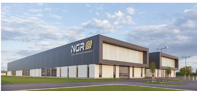
The new energy-efficient NGR plant in Feldkirchen/ Donau (Austria) offers sufficient space for innovations and individual solutions to further advance the recycling economy (Photo © Kurt Hörbst)
