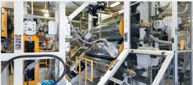
J-stack configuration featuring roll-skewing and electric gap adjustment under full hydraulic load
